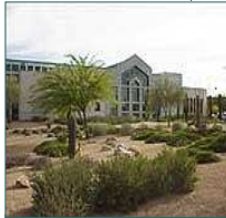
West Charleston Library, Las Vegas-Clark County Library District
